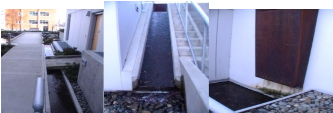
Concrete Runnels flow into creek.
