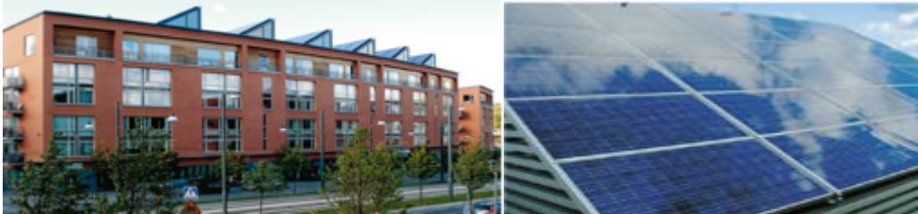
Hammarby Sjolstad Solar panels that exploit the sun's heat and use it to heat the hot water supply have been installed on many roofs. The solar panels shown in the picture are sufficient to meet half of the building's annual hot water requirement. Courtesy Hammarby Sjolstad
