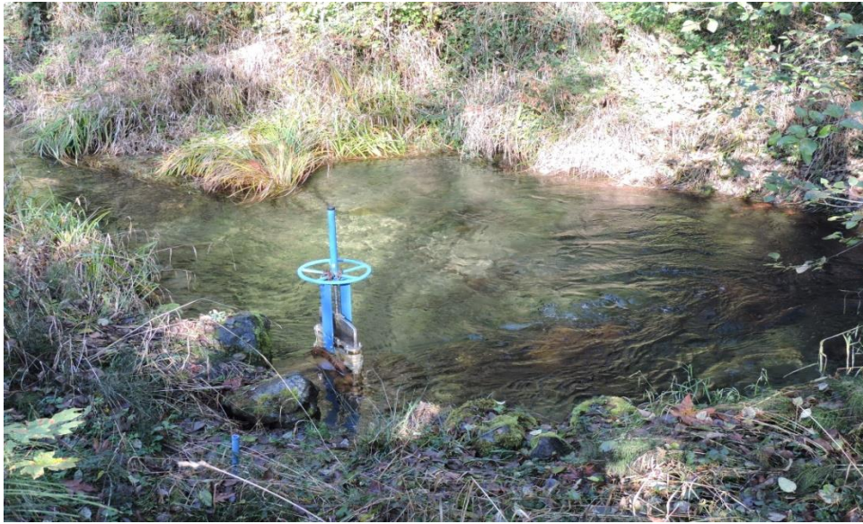
Site 1- Picture of pipe and control valve for flow located at the top end of the side channel. Picture taken on November 18, 2015.
