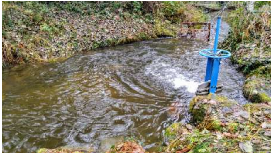
Photograph 1.2. Site 1 looking downstream on the C.W. Young Channel and at one of two blue manual water flow control valves located here and a debris screen placed mid-channel. From the water flow control valve in the photo, the second valve is located upstream approximately 15 m. Oncorhynchus Keta O. kisutch were observed swimming here. Photo by Tamara Stauffert, 31 October 2016.
