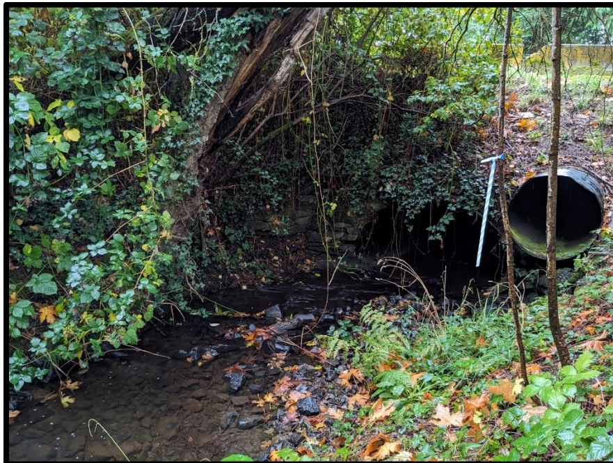
Figure 8. Site 4, looking downstream. Note the two culverts in place to control varying levels of flow (Taken on October 10, 2023).
