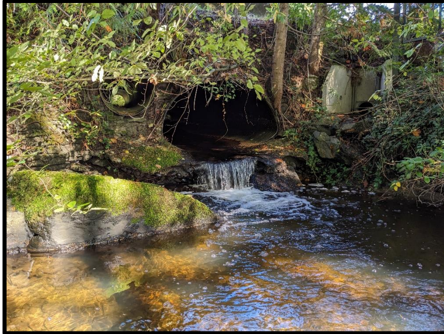
Figure 9. The downstream end of the culvert from site 4, with a drop-off that prevents pacific salmon from entering into Cottle Creek (Taken on October 11, 2023).
