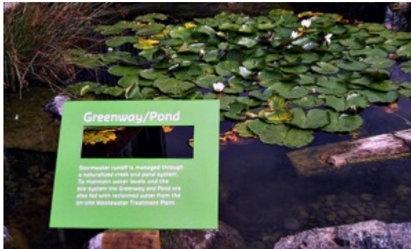
Retention Pond, Courtesy Dockside
