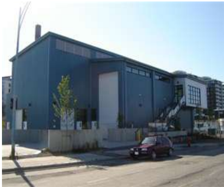
Biomass Plant, Courtesy Dockside
