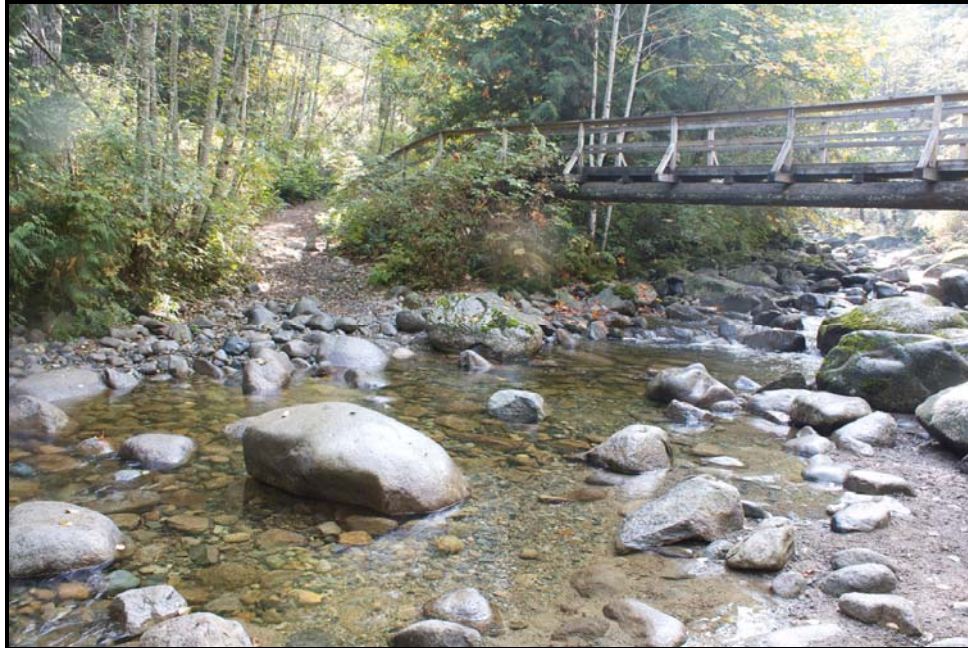
Photo 1. Upstream view of Holland Creek at station 1, with wooden bridge visible in background.
