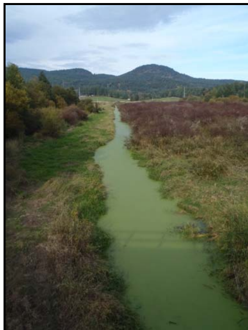
Photo 4. Upstream view of Richards Creek at the Herd Road Bridge (station 4).
