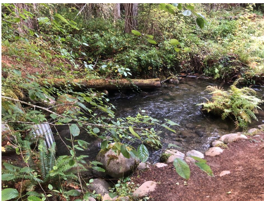
Figure 2: Site #2 of the C.W Young Channel, facing downstream of the culvert.
