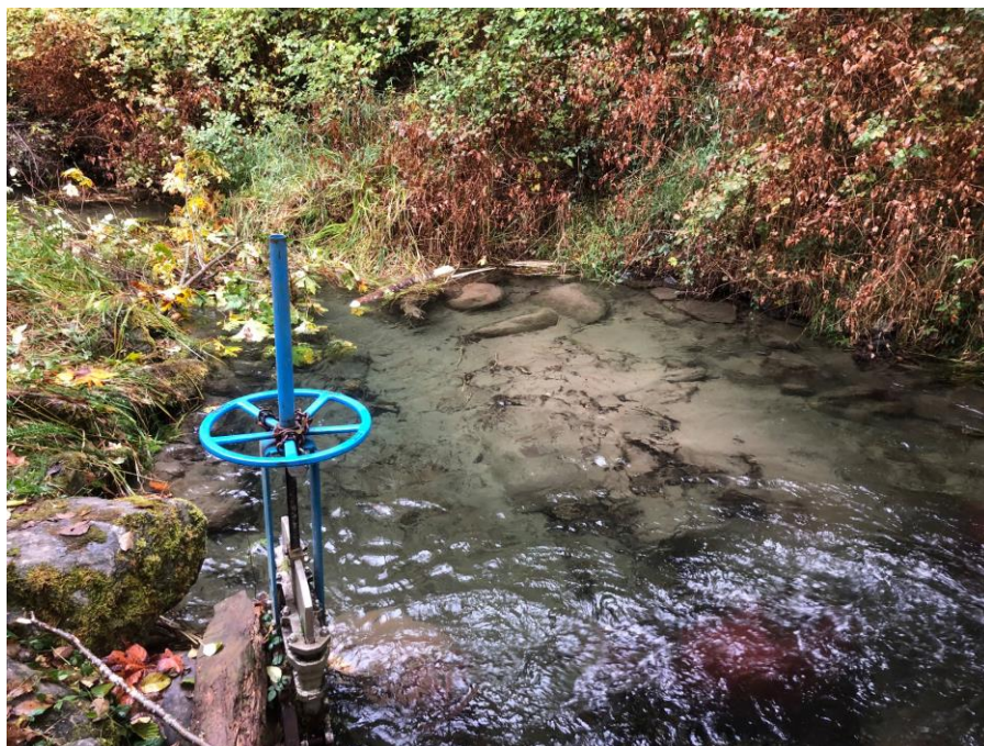
Figure 1: Site #1 of the C.W Young Channel. Note the beginnings of a beaver dam being constructed upstream of the outlet during the first sampling event.
