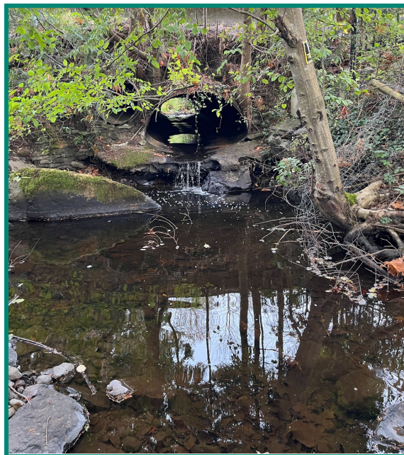
Figure 28. Image of downstream view of Cottle Creek (October 26, 2022).
