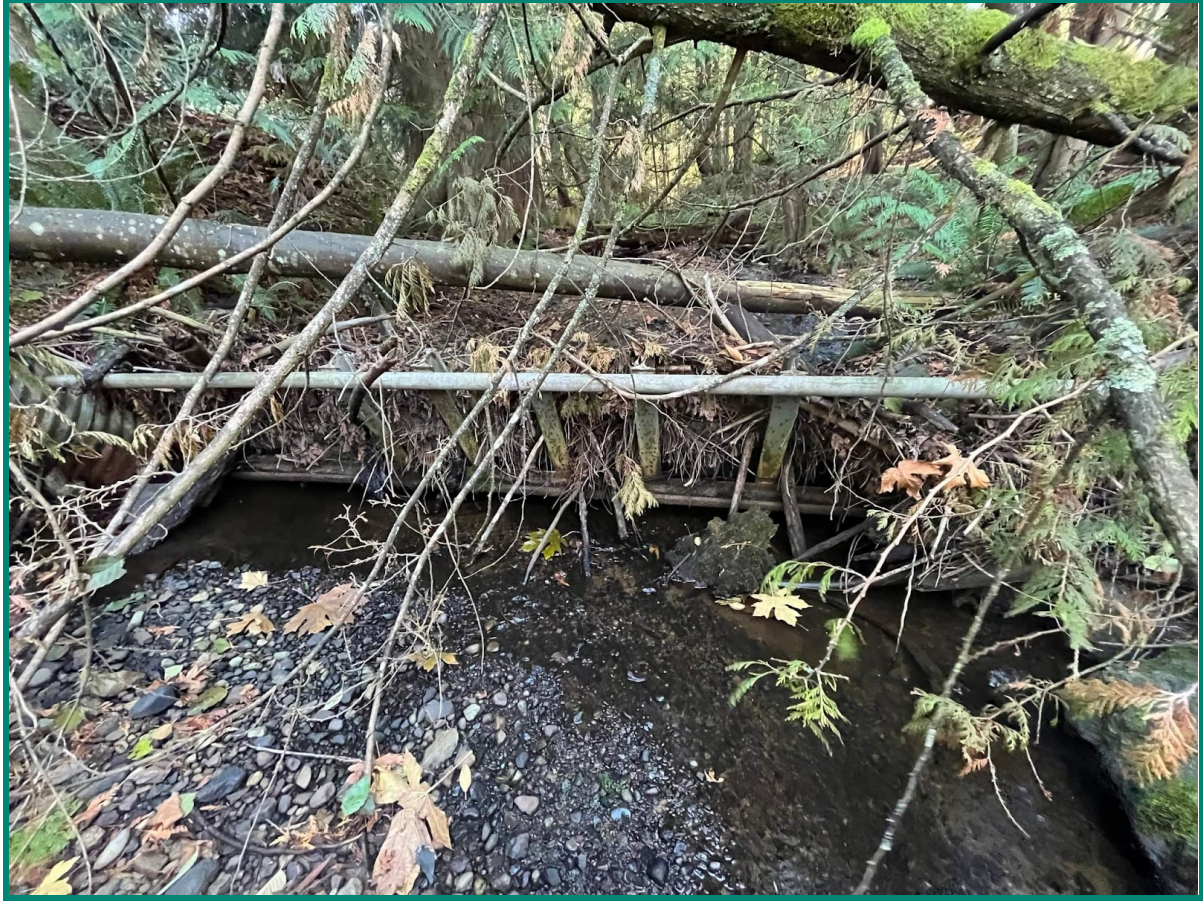
Figure 18. Woody debris culvert sieve acting as a fish passage barrier at Site 1.
