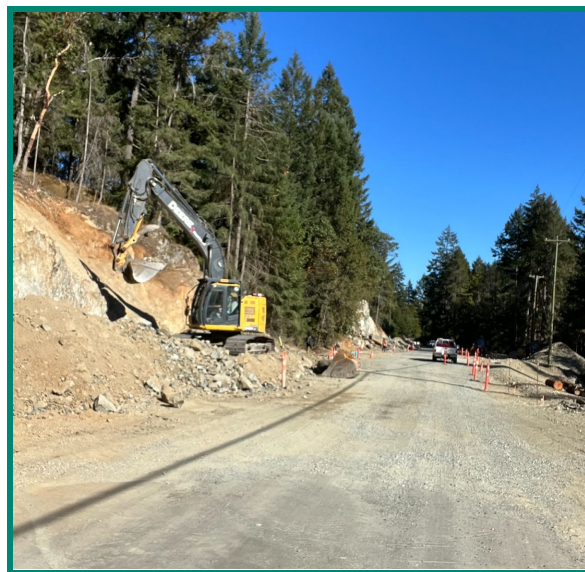
Figure 20. Road Work on Rock City Road, October 12, 2022.
