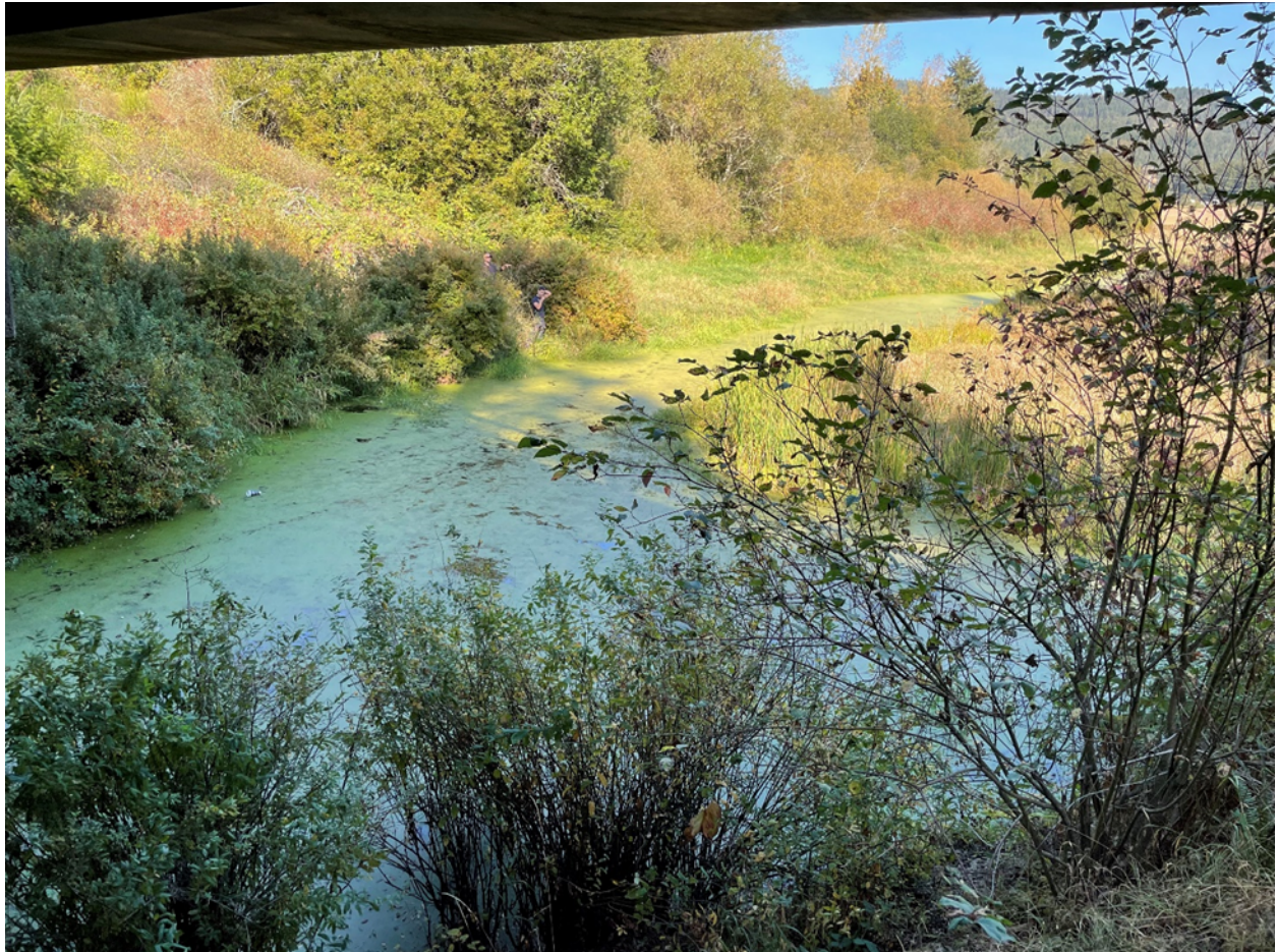
Figure 7: Site 4 underneath Herd Road Bridge with visibly green water (Bell 2022)
